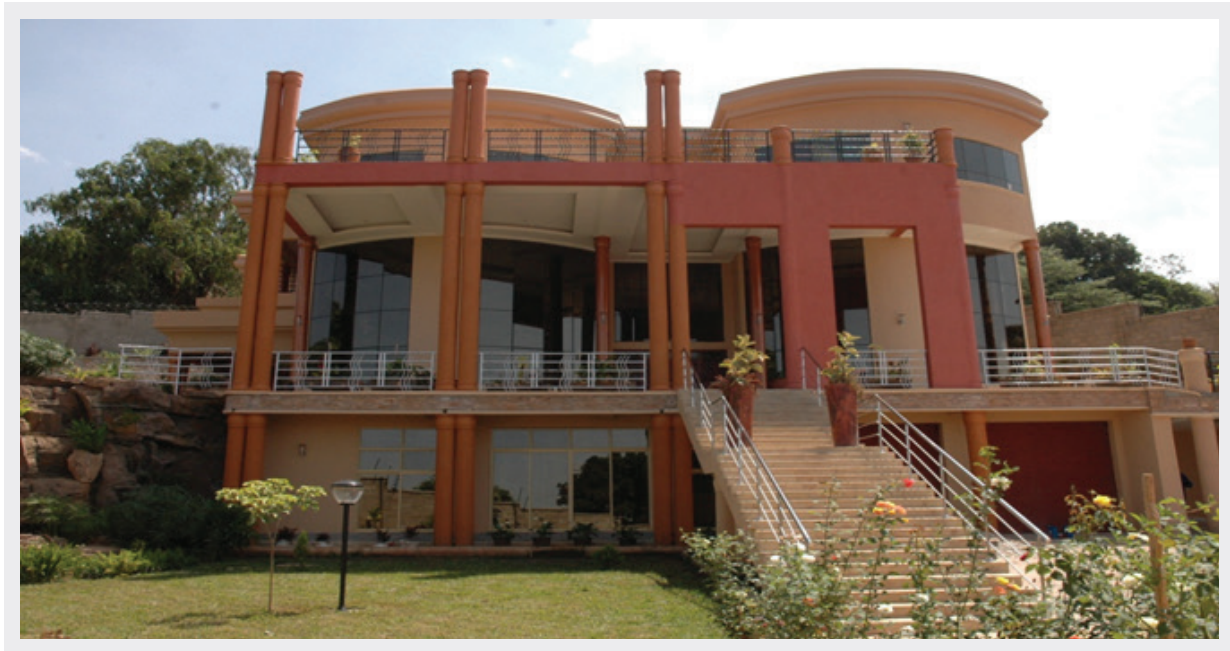
Residential house at Mbuya constructed by Aswangah construction services front view
