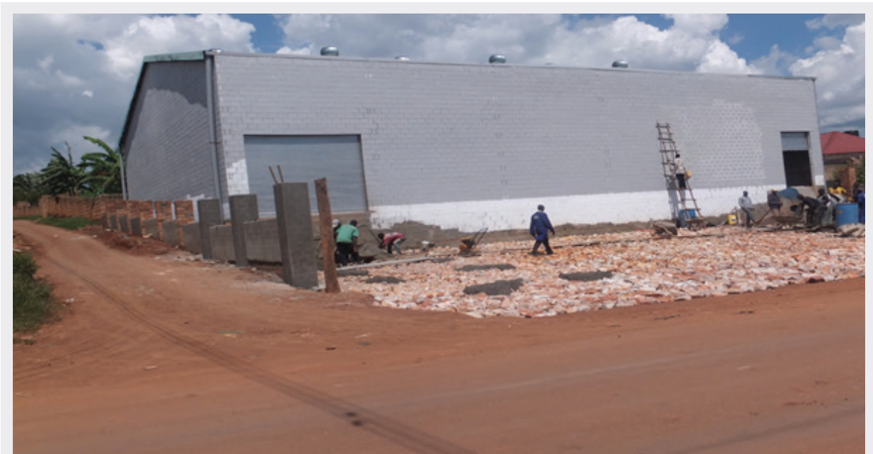
| Ware House Constructed at Kira T/Council For Daks Couriers. |
