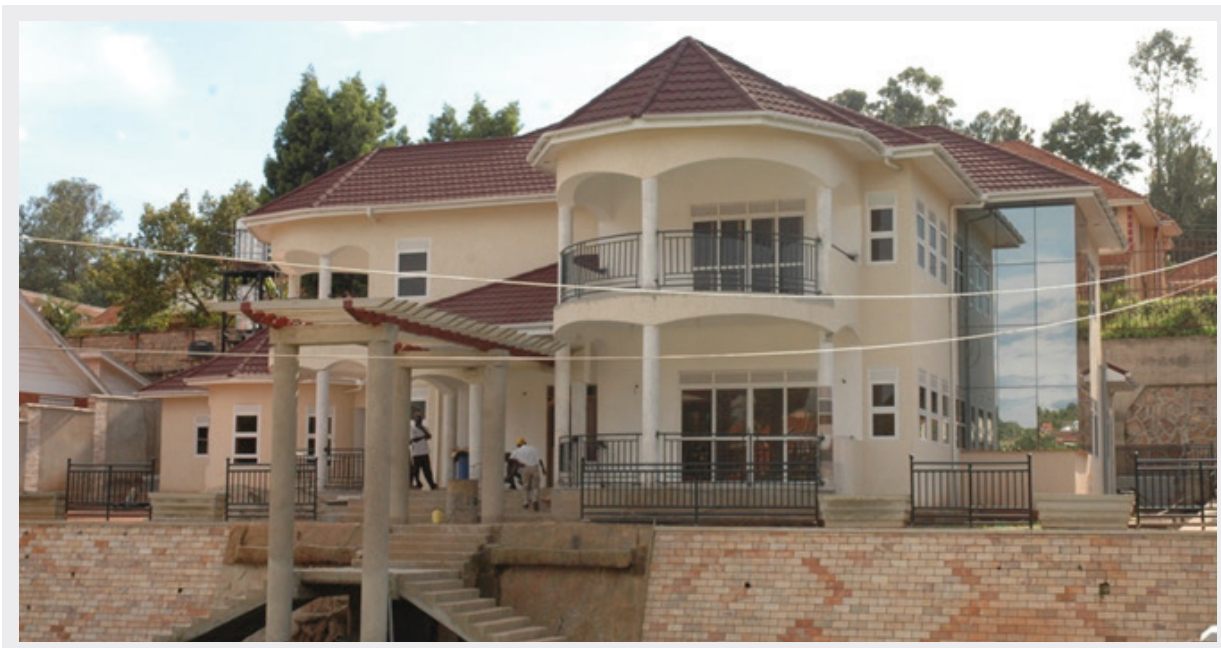
Residential building in Naguru for Pexy Investments after construction
