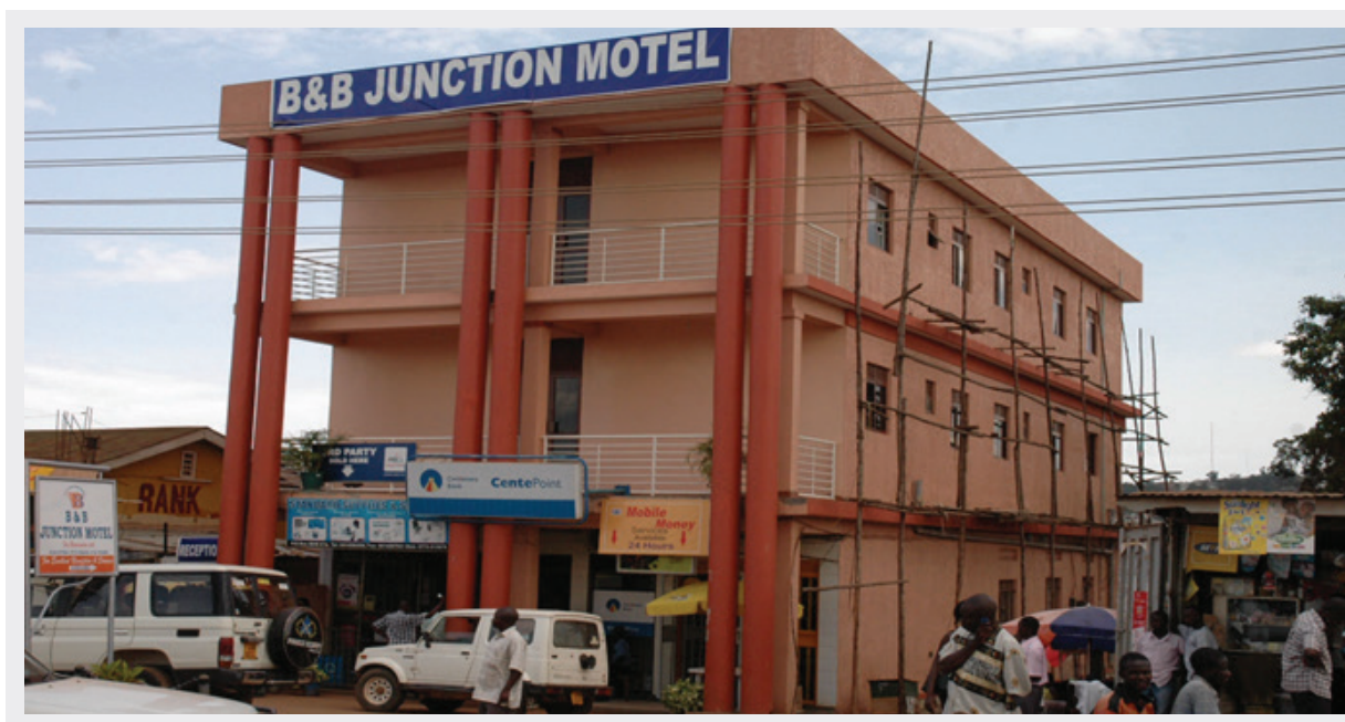
B&B Motel in Ntinda – KAMPALA, Modified by Aswangah construction services
