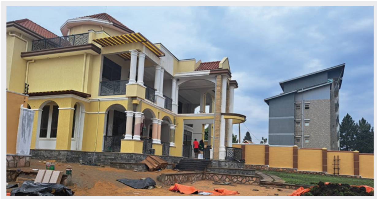
Kyanja Residential development – after construction
