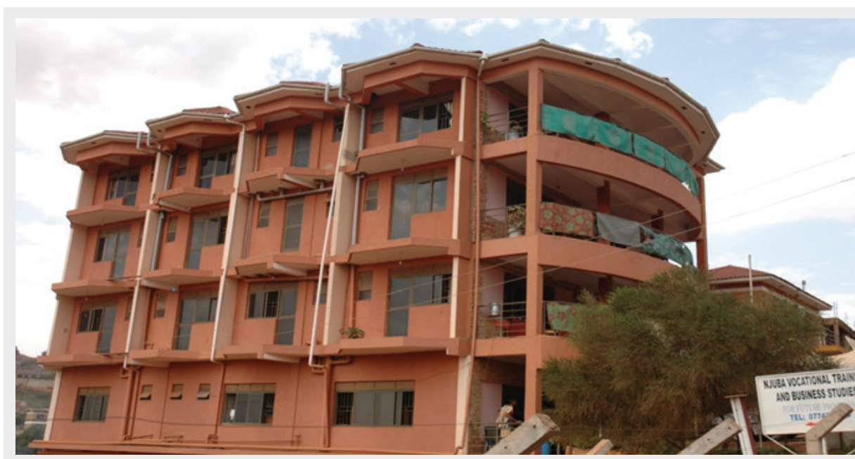
Satelite Hotel in Kisasi – Kyanja road constructed by Aswangah construction services
