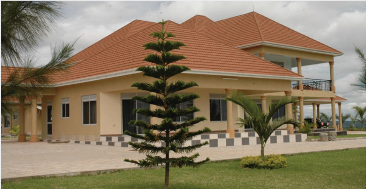
Residential house along Mityana road constructed by Aswangah construction services
