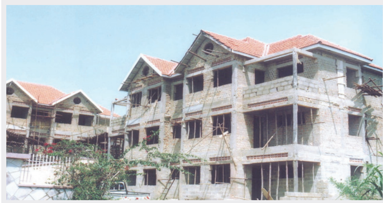
Residential Apartment at Munyonyo constructed by Aswangah construction services under construction
