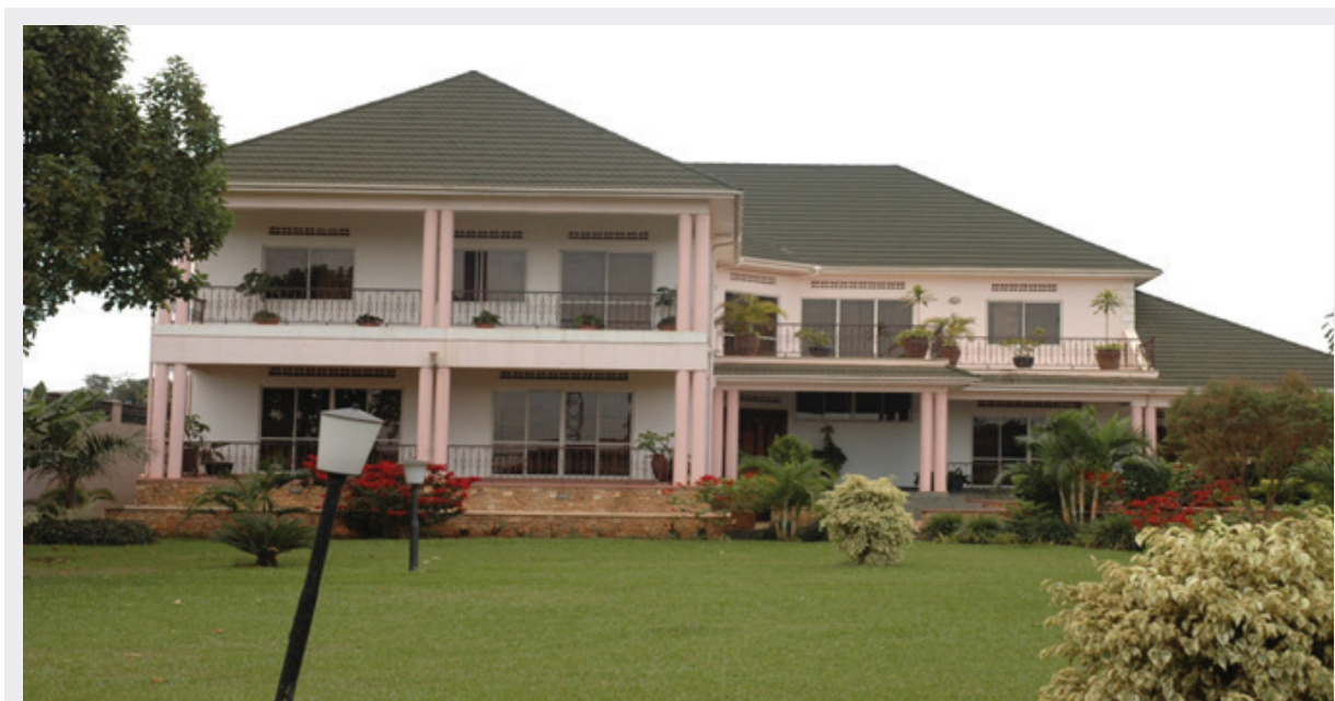
Construction of a residential house in bukoto Client: Private developer
